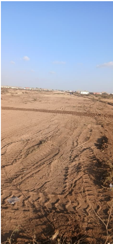
Photo 1 — Opened arterial corridor, Sector A
