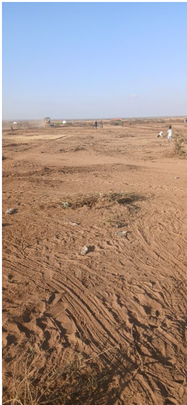
Photo 2 — Site clearing works in progress
