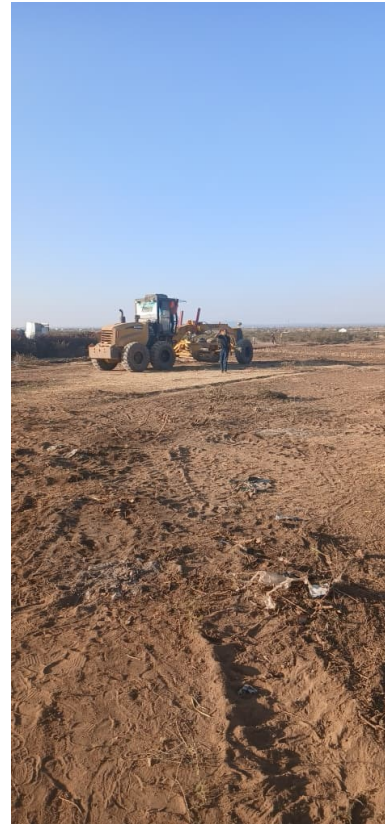
Photo 4 — Grader deployed on the arterial road corridor
