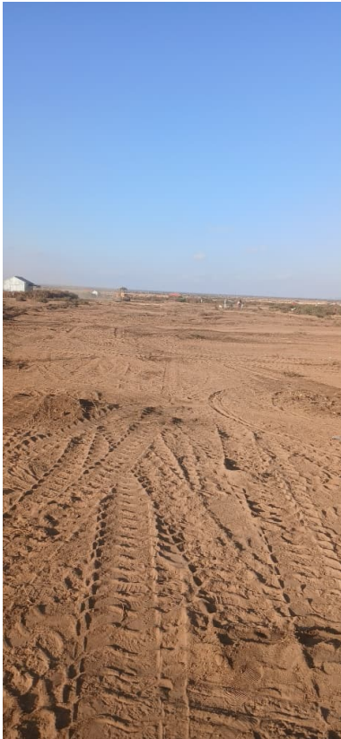
Photo 3 — Cleared right-of-way looking toward built-up area
